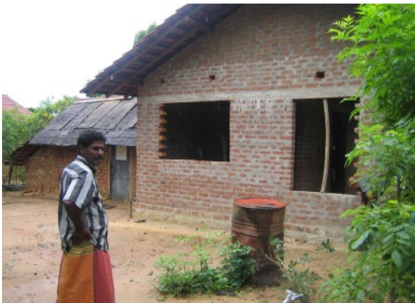
The partially built house – but the widow lives in the adjoining shack
